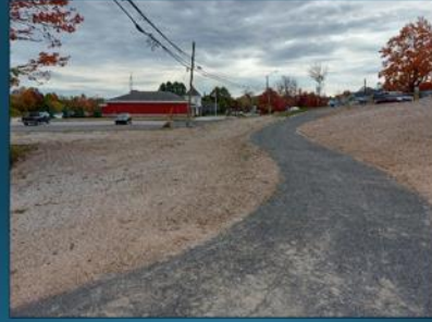
Looking south to Park 'n Ride parking lot and Berwick Fire House
