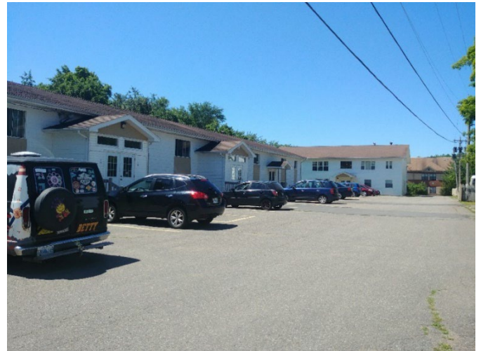
Picture 3 - Buildings on adjacent property to the north
